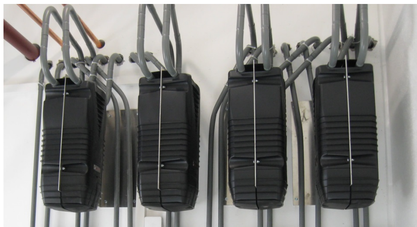
VULCANs installed back to back
