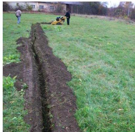
Picture 5: The ground trencher and the possibilities
