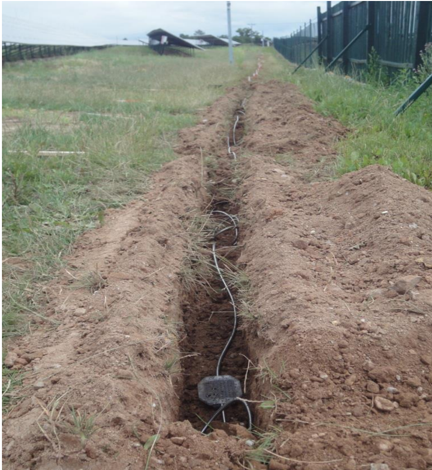
Picture 4: The trench made by the ground motor trencher
