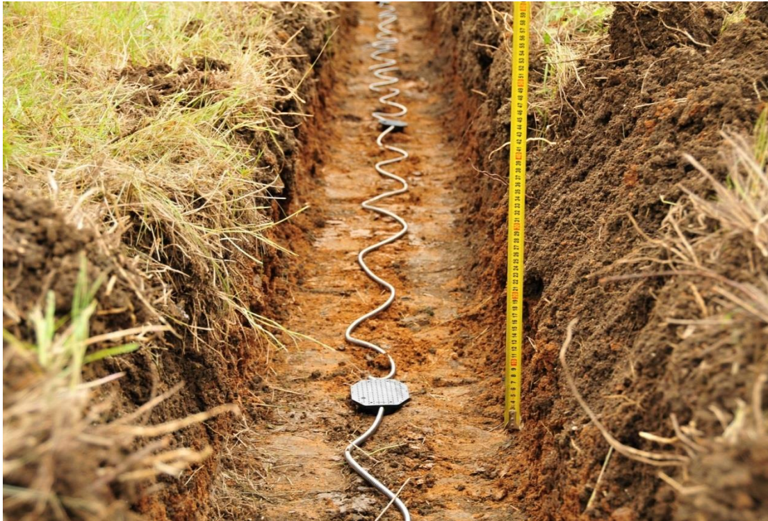
Picture 2: The cable ripple (the trench made by the excavator)
