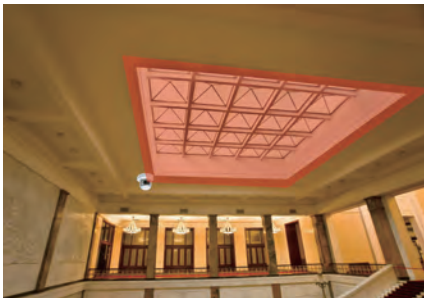
Skylight protection at Public facility / Warehouse
